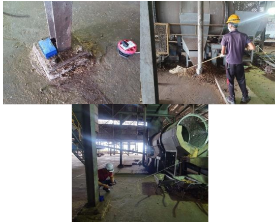
Fig 9: Location of low-cost device at critical location
