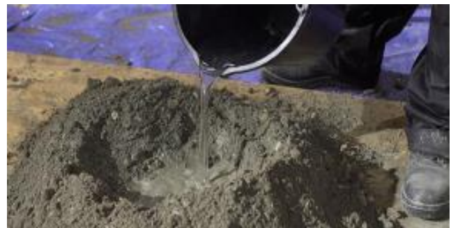
Fig. 1 Preparation of concrete
