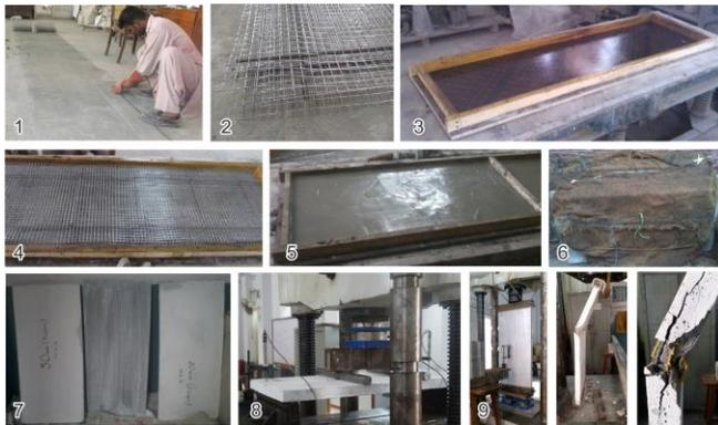
**Fig 3: Method of casting ferrocement slabs**
