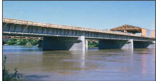
Fig. 4.1 The Taylor Bridge during construction.
