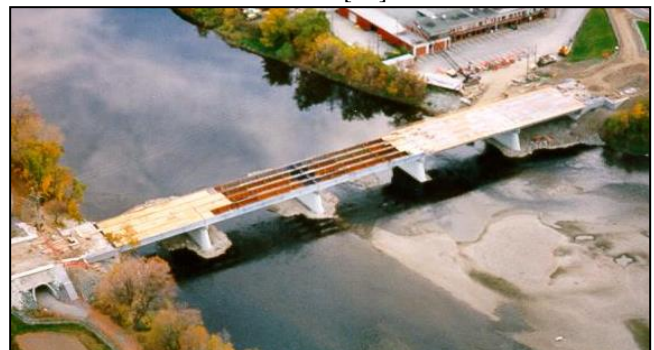
Fig. 4.2. the Joffre Bridge
