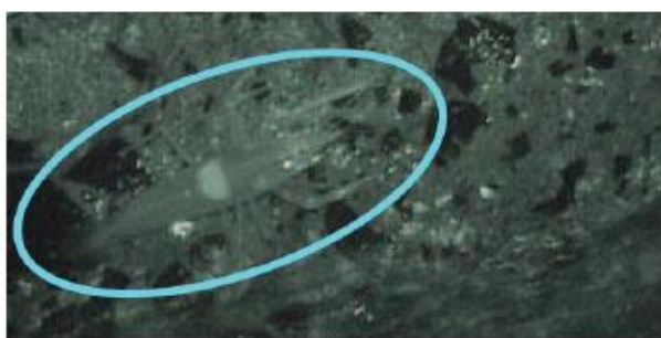
Figure 5: Entry of sediment causes the inefficiency of the fish way
