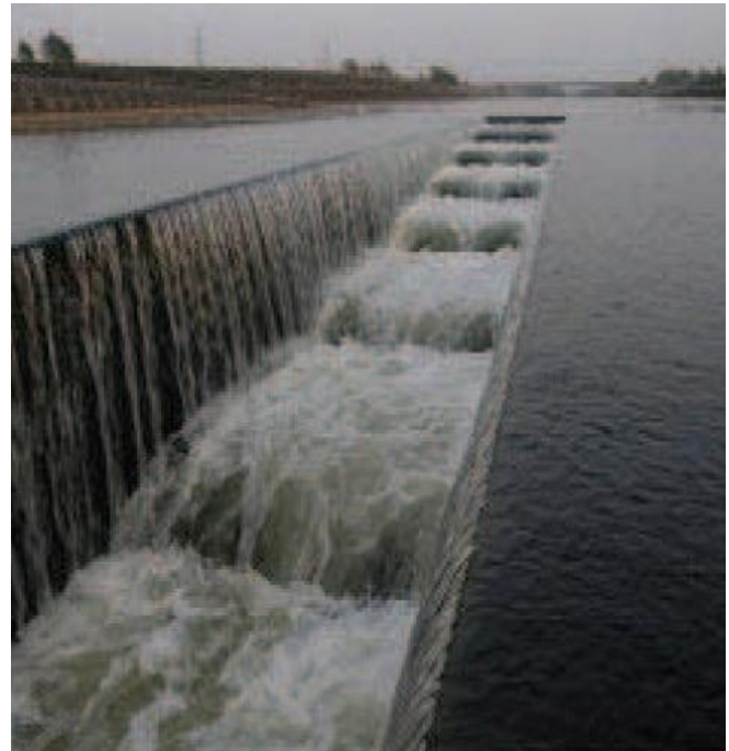
Figure 2: Improper flow conditions in small floods at the upstream of the fish way (type of Pool-weir)
