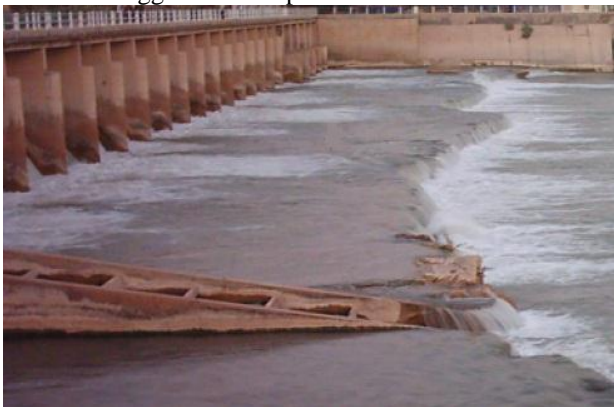
Figure 1: The downstream conditions of the fish way constructed on Karkheh dam
