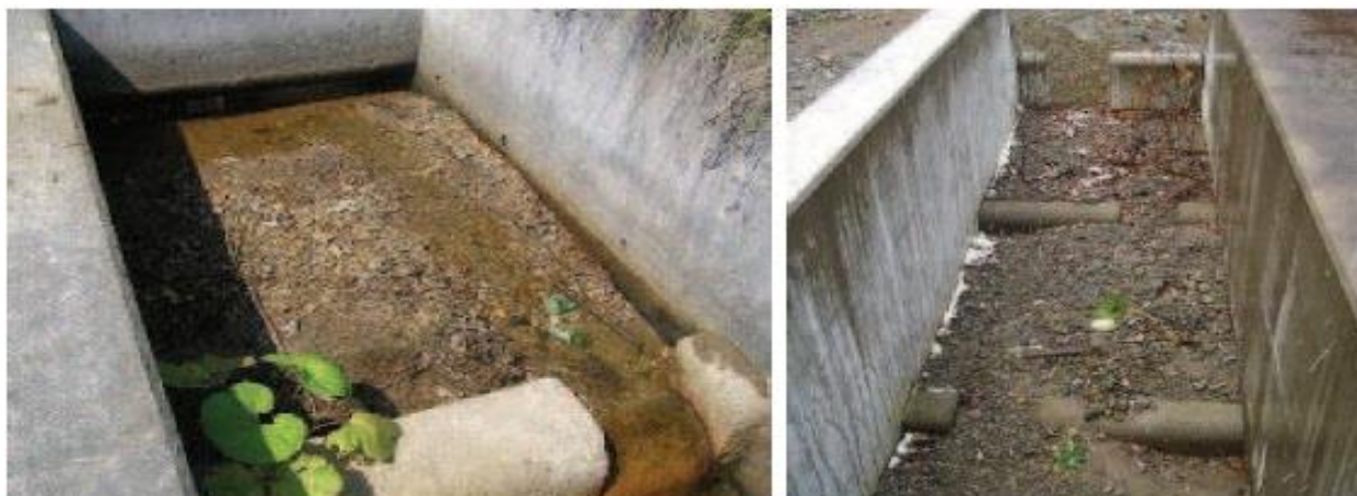
Figure 5: Entry of sediment causes the inefficiency of the fish way
