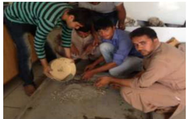
Fig.1: Preparation of concrete mix
