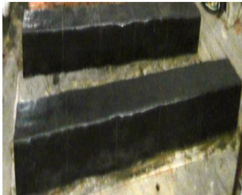
Fig.3: Application of CFRP wrap in U-shape
