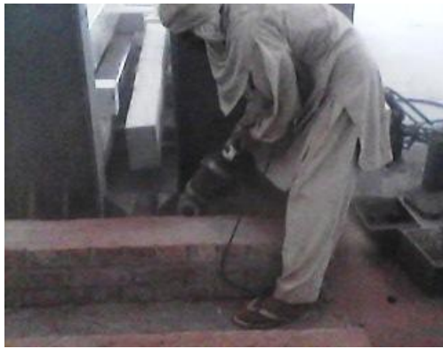
Fig.2: Grinding of Masonry beams
