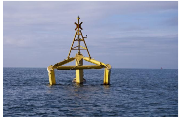
Figure 9b: E35 successfully installed into Sanda Sound [36] Verdant Power Ltd.
