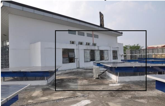
Figure 6: Some PV arrays too close to the building
