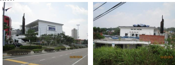
Figure 1 : Maahad Tahfiz Negeri Johor, Nong Chik (L) and the location of the PV panel on the roof (R)
