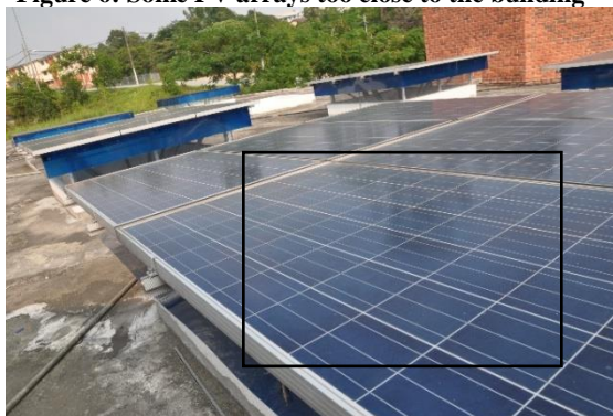
Figure 7: The PV surface needs regular cleaning calculation simulation ( \eta sim) and the real PV system efficiency ( \eta real). It was also found that some PV panel surfaces needed cleaning because of dirty spots (figure 7).
