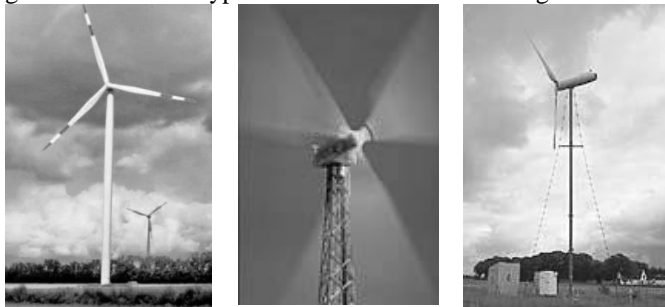
(a) Tubular Steel Tower (b) Lattice Tower (c) Guyed Pole Tower
