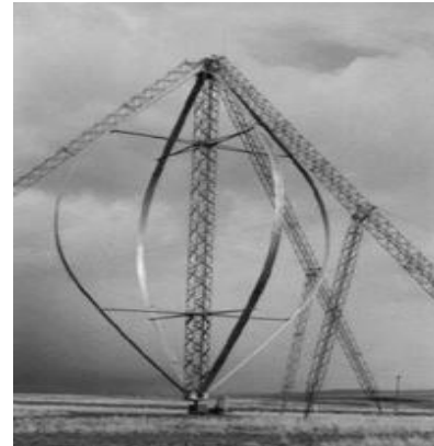
Fig. 14: A Curved Blade Rotor with Four Blades
