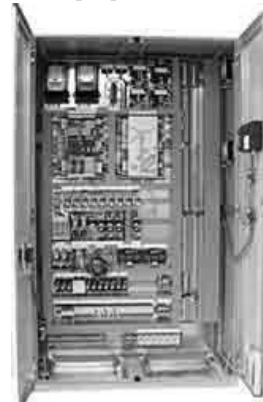
Fig. 10: An Electronic Wind Turbine Controller
