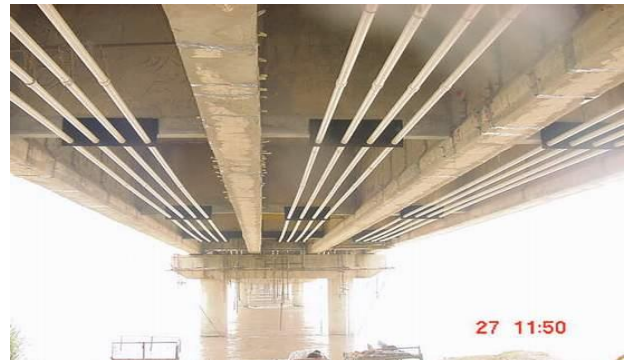
Figure 10 External Post-Tensioning
