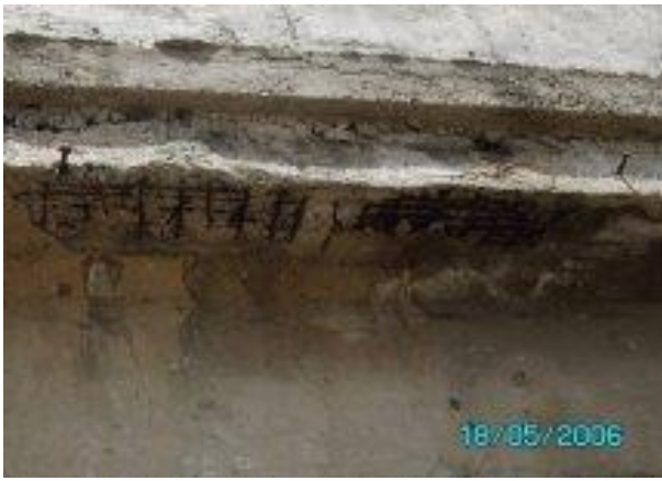
Figure 1 Exposed Reinforcement
