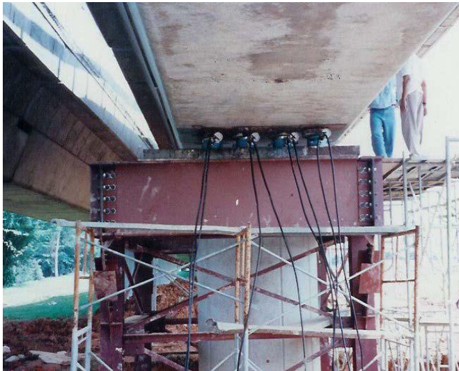
Figure 5 Arrangement for replacement of a mechanical pot bearing of a bridge
