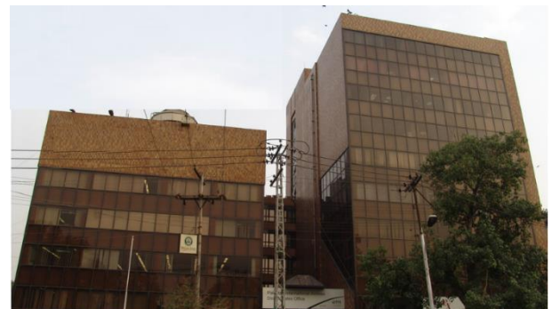
Fig. 6 The selected Multi Storeys Building
