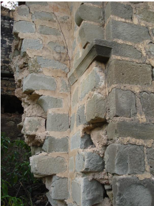
Fig. 6. View of Elevation
