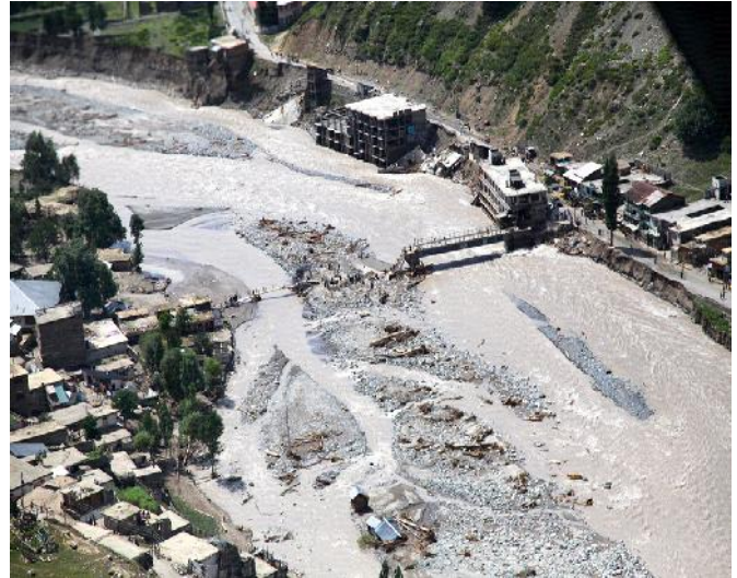
Fig. 2. Washed out bridge & buildings (constructed in river course) by the flood in Ghazi, August 5, 2010 (Reuter's/Horace Murray/U.S. Army)
