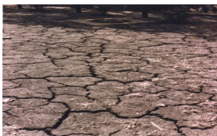
Fig. 2: Polygonal pattern of surface cracks in the dry season.
