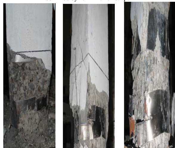
Fig 20: Failure of CSP2
