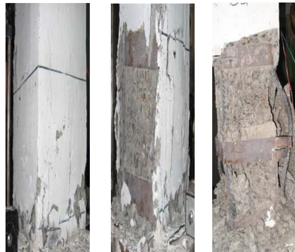
Fig 17: Stepwise Failure of CSP1
